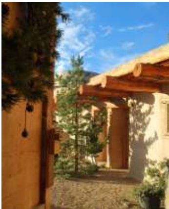
Over 5,000 logs from the mountains and some local backyards were peeled by hand for vigas and latias.
